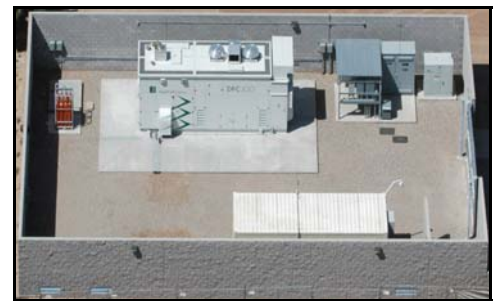
Fuel Cell Energy DFC300A Commercial Fuel Cell System
